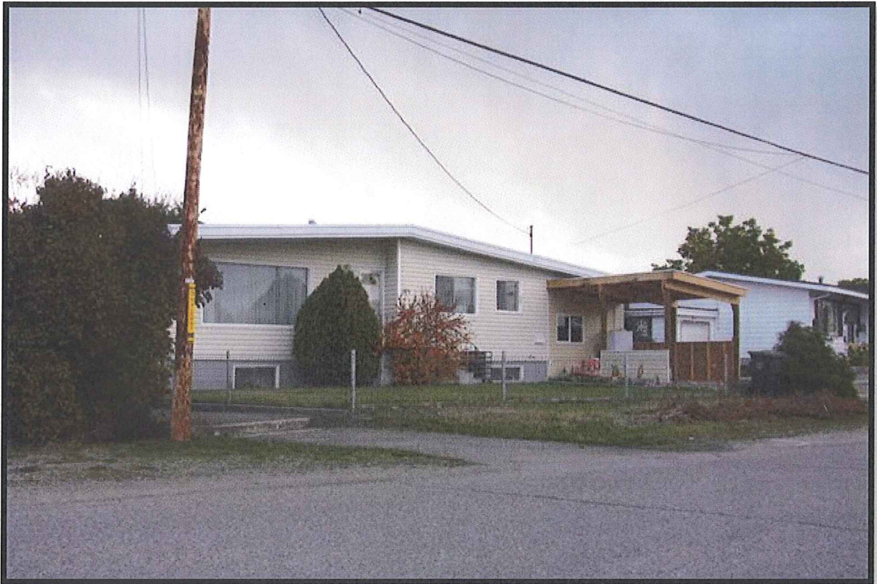
DVP11-0178 - 185 Robson Road East Photos of carport under-construction
